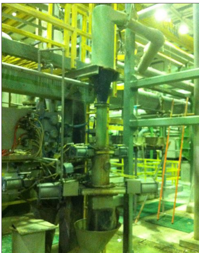
Figure 22 Single heavy-duty metal vortex cleaner
